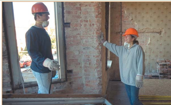
Building Brighter Tomorrows activities include refurbishing shelters and homes.
